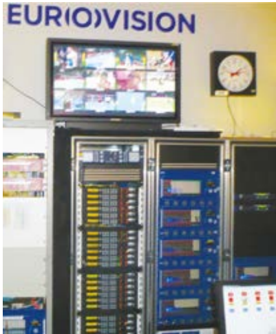
Phoenix audio codec system at London 2012 for Eurovision. 24 codecs pool working together with another 48 units distributed in different countries.
