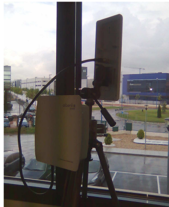
Detail of a WiMAX base station and associated antenna on a tripod
