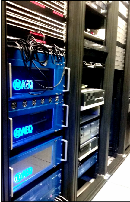
Barcelona Central Control Room Matrix & Codecs
